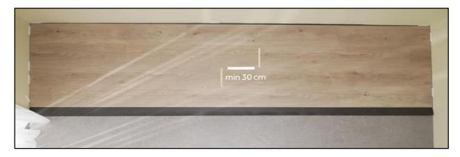
Step on the rows that have already been installed, this will make further installation easier.
