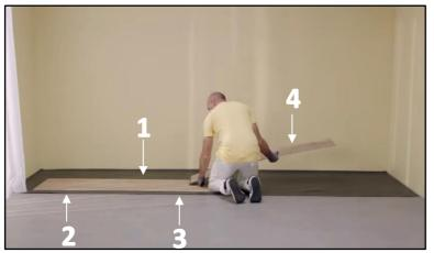
4. Place a fourth complete plank (n°4), at an angle of +30 degrees, on the long side with the tongue in the groove of the first board (n°1) of the first row and lower it. A narrow gap is now visible between board n°4 and board n°3. To do this, lift board n°4 at an angle of +30 degrees and pull it with the tongue into the groove of board n°3.
