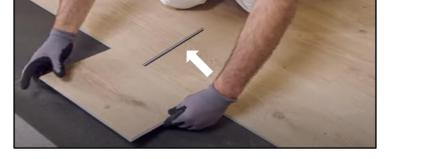
5. Repeat actions 3 and 4 until you reach the end of the first two rows. Then slide the whole thing nicely against the wall. Use spacers to respect the expansion gap of 5 mm. Leave these blocks in place during the entire installation for an optimal and linear straight result.
