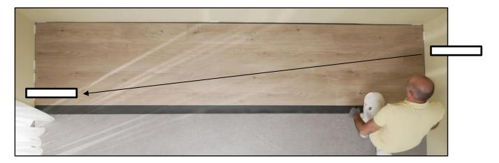
Always ensure that the ends of the planks in two successive rows are the same and that the distance between the short ends is at least 30 cm.
