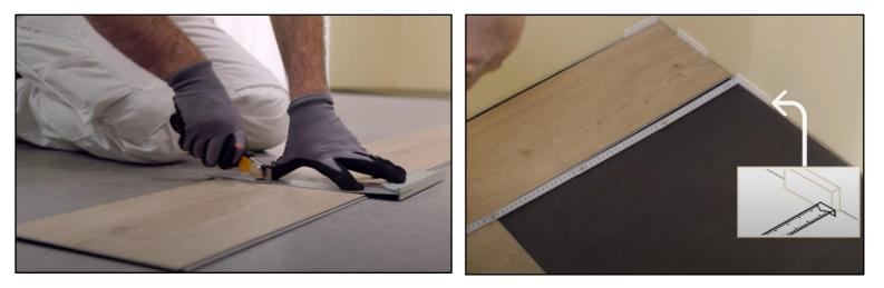
7. From the third row onwards, place the planks row by row. Make sure that you place enough spacers in the expansion joints so that the floor does not shift. Use a varying mix of decors and planks from different packs.
