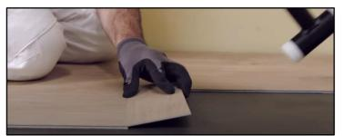
(Advice) Alternative assembly method: A floor board can also be clicked together with the long side first and then with the short side into the other board. For this last step you can use a tapping block. This can be a short piece of cutting waste that you click onto the plank to be installed. Never hit the click connection directly with a hammer and make sure that the floor is completely fixed! To guide the plank better, you can click a short piece into the next row for guidance.
